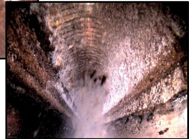
Surface Damage Reinforcement Visible (SRV)
