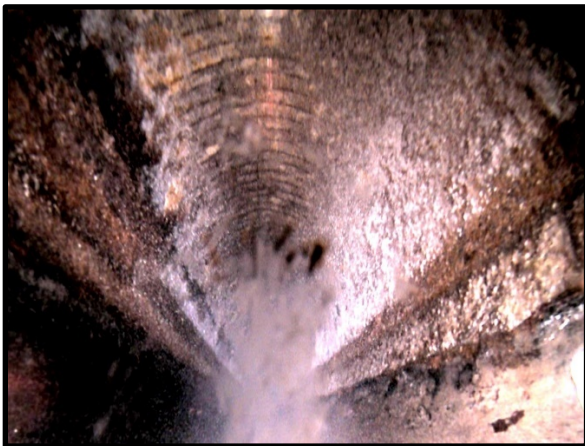
Figure 6 Surface Damage Reinforcement Visible (SRV) Pipe Segment: SL7660 at 6.6 ft
