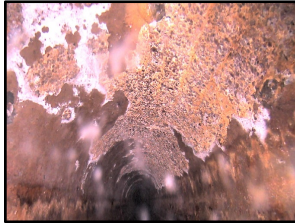
Figure 5 Surface Damage Aggregate Projecting (SAP) Pipe Segment: SL11054 at 271.4 ft
