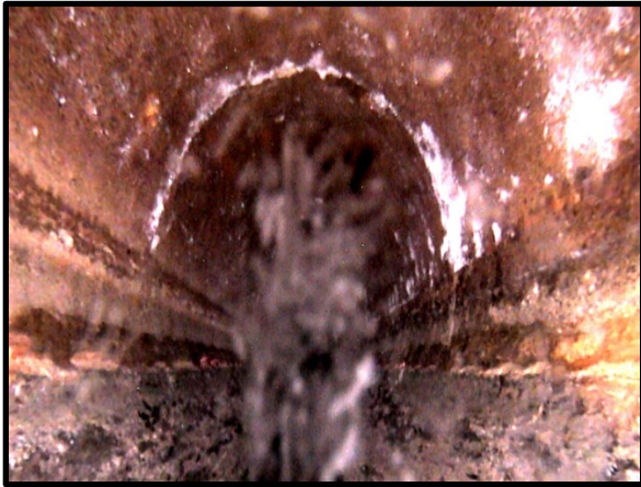
Figure 4 Surface Damage Aggregate Visible (SAV) Pipe Segment: SL2477 at 0.3 ft
